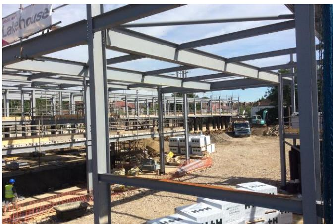
The pace of progress on the new school building in the last few months has been amazing. At the time of the last newsletter in April the building foundations were still being dug and laid. Since then the steel framework has been completed and the floors have been laid on both the ground and first floor with brickwork reaching to the first floor. You can now clearly make out the size and scale of the building and recognise individual rooms and spaces.
